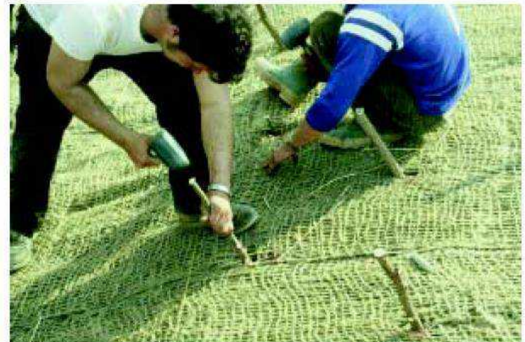
Live staking. Robbin Sotir & Associates
