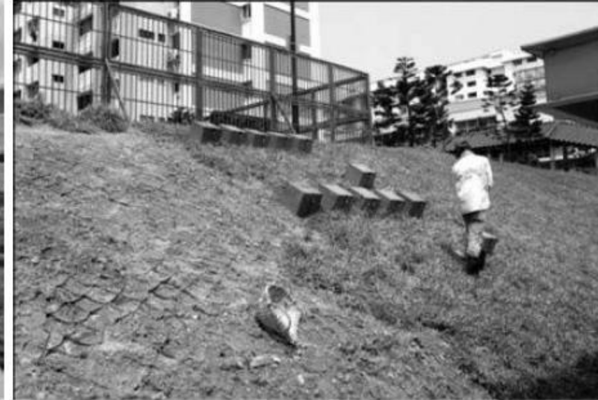
(c) Grass planting on slope surface after placement of the top soil on top of the capillary barrier (boxes on the slope surface are tensiometers)
