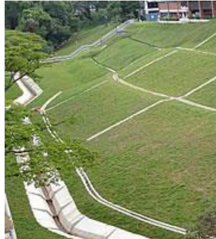
(b) Slope with horizontal drain
