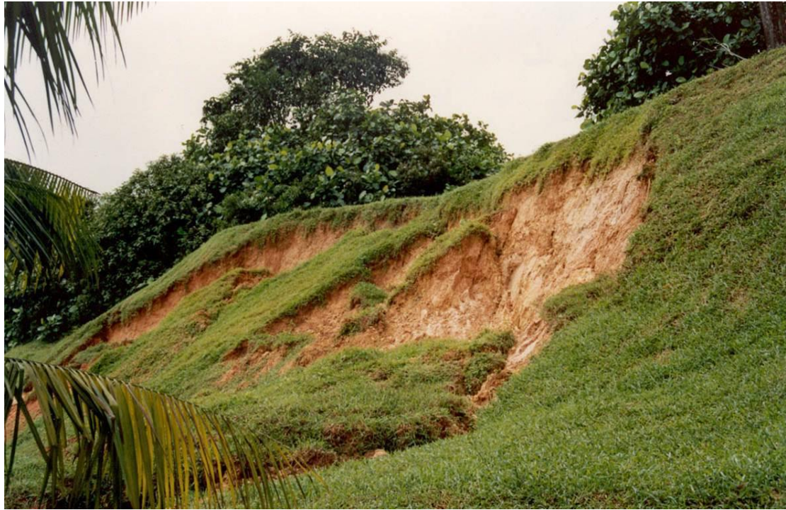
Nature and form of a few slope failures (out of 20 slope failures) on 26 February 1995 in Nanyang Technological University Campus (sedimentary Jurong formation), (Rahardjo et al., 2012)
