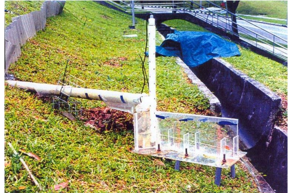
Field installation of a flume with water depth probe for runoff measurement at NTU-CSE slope, (Tsaparas et al., 2003)
