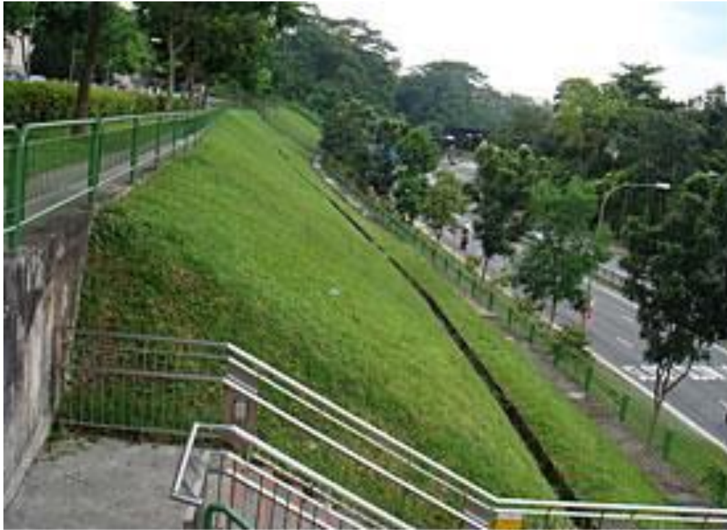
(a) Slope with vertical and horizontal drain
