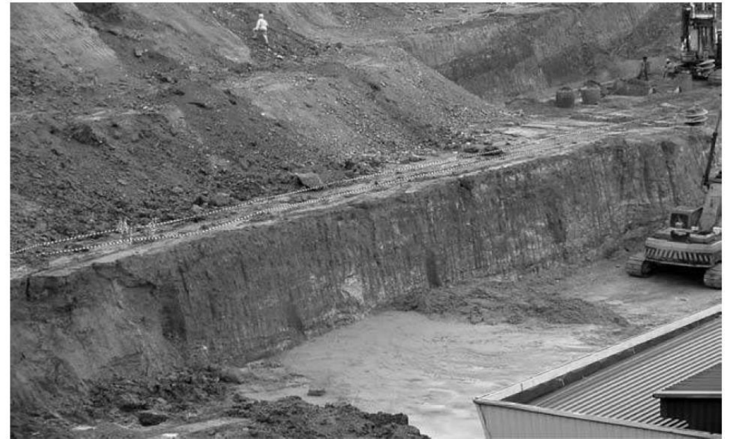
Profiles of residual soil of the sedimentary Jurong formation ( Rahardjo et al., 2012 )
